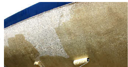
Applying Safeguard LVP
