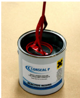
Mix thoroughly with a spiral mixer used in a cordless drill
